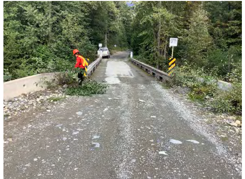
Left Bank Abutment when facing downstream
