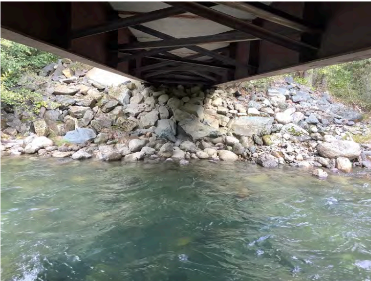
Right Bank Abutment when facing downstream
